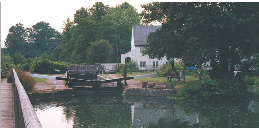
• Stort Valley lock at Twyfordbury (P. Shears)
